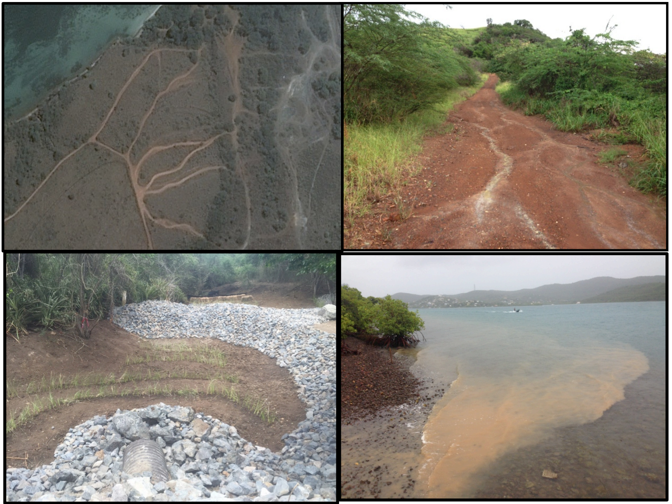
Figure 12. Clockwise from top left: Dirt roads in Los Pozos near Combate, a significant source of sediment to coastal waters, (right) example of surface rills conveyance over the road surface creating erosion and resulting in fine sediment losses, bottom right sediment reaching coastal waters; bottom left: recently constructed sediment trap in Cabo Rojo to capture sediment before it enters Boquerón Bay
