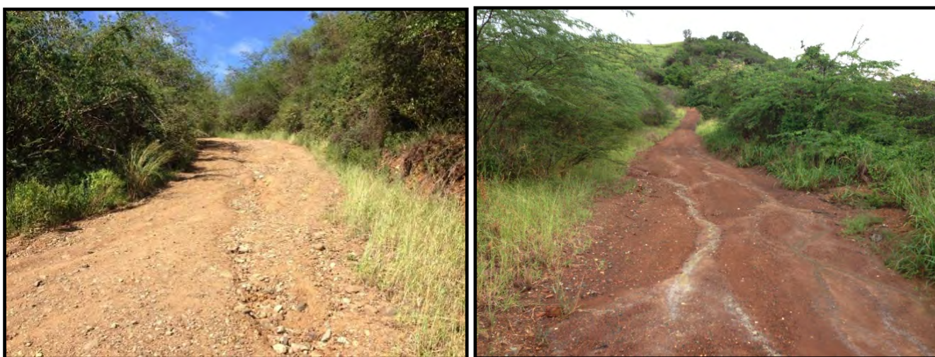
Figure 18. Dirt roads as a source of sediment (note the surface runoff over the roads creating erosion and resulting in fine sediment losses)
