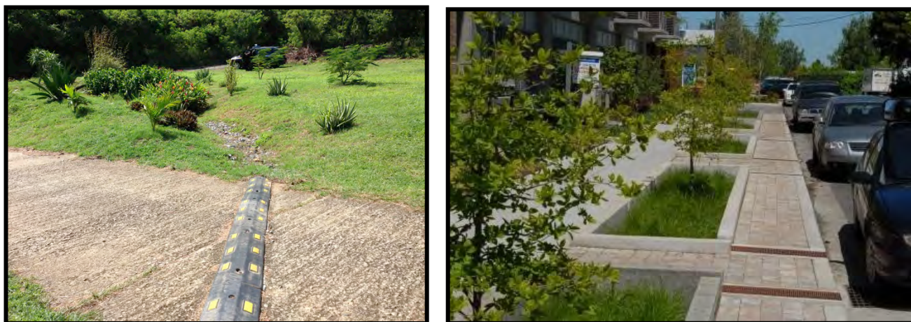
Figure 16. Rain garden from St. Croix and streetscape biofilters from Santa Monica, CA
